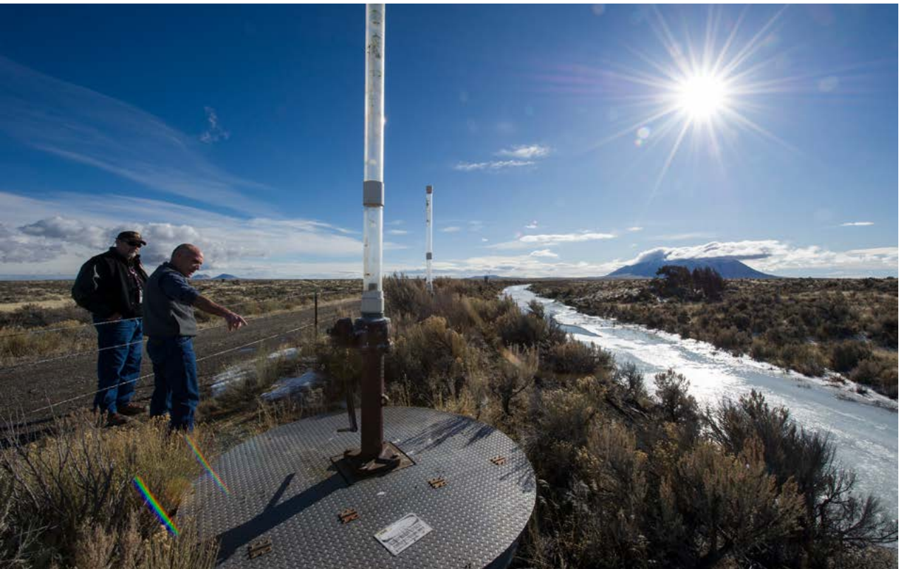
DOE Facility Representative Steve Karns listens as Steve Christensen describes operation of the diversion gates. The river flow at the right has been diverted to the south from its natural course.
