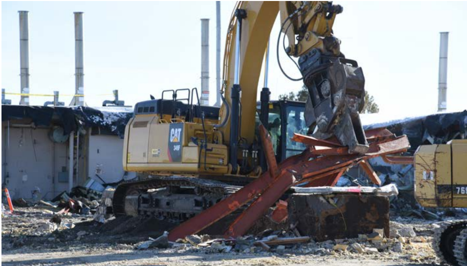
Jerry Cloward uses a processor arm to move structural steel to a separate pile for recycling.
